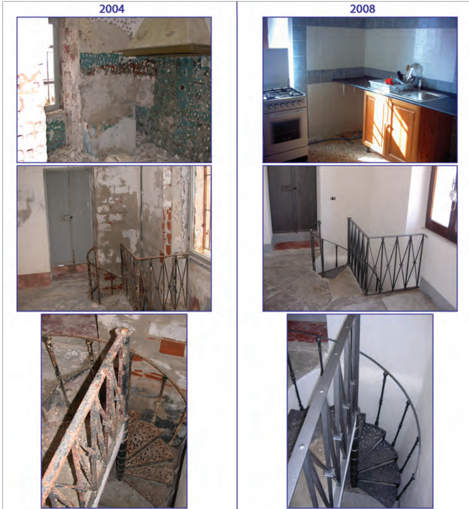
Figure 5 - Punta Sardegna Lighthouse, inside before and after renovation.
