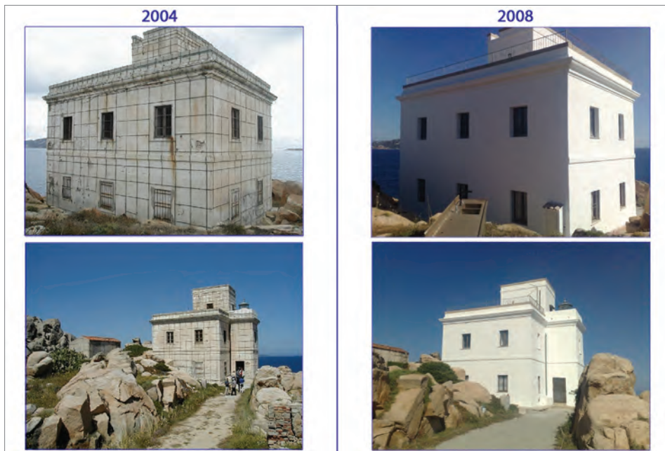
Figure 4 - Punta Sardegna Lighthouse, operating headquarters for OCEANS and the “Centro Transfrontaliero per lo Studio della Dinamica dei Litorali” (cross-border centre for the study of coastal dynamics), before and after renovation.
