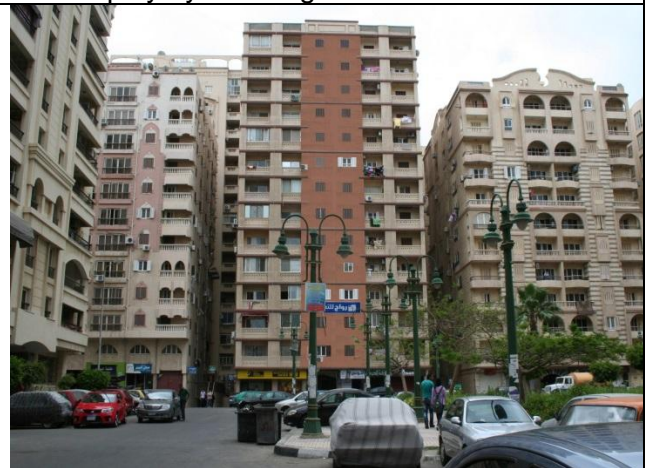
(D) Coloured polycrystalline glasses in balconies and a solar shading PV technology
