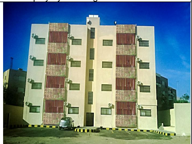
(D) Coloured polycrystalline glasses in balconies and a solar shading PV technology
