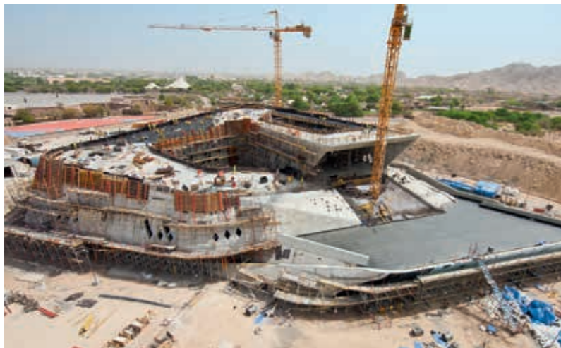
Fig 2 Desert learning center construction site, Al Ain - Abu Dhabi
