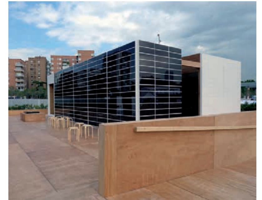
Fig 3 Ventilated PV façade. Built for Solar Decathlon Europe 2010
