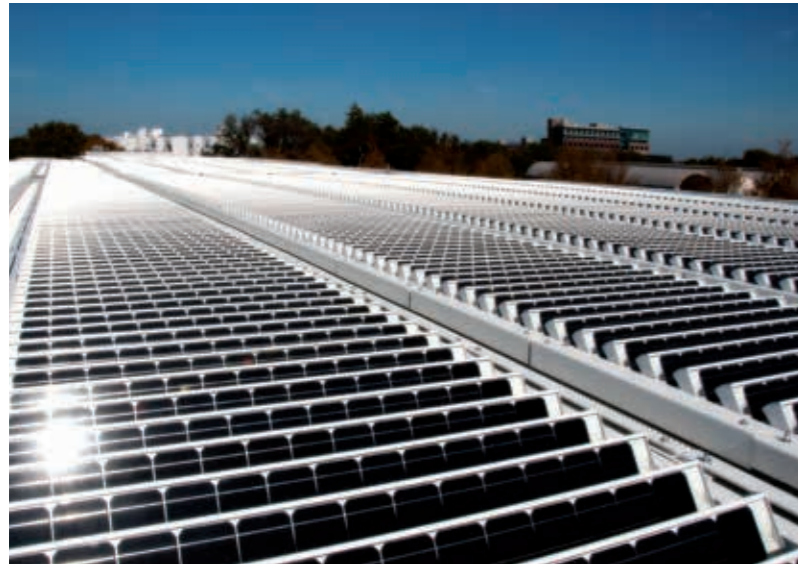
Fig 17 New Pavillon at Kimbell Museum, USA. Roof.
