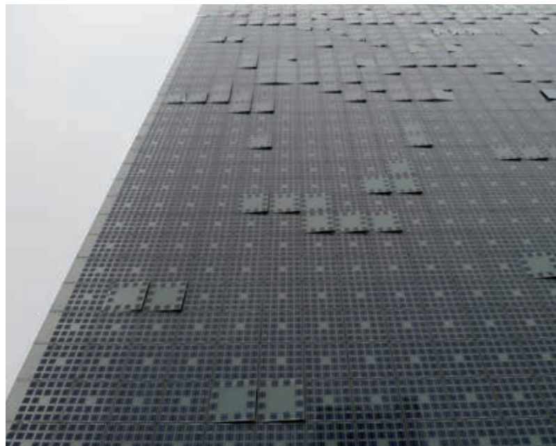
Fig 4a, 4b Curtain wall PV system
